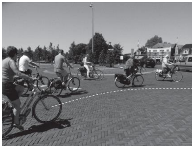
Figure 2. Sneek (Prins Hendrikkade). A dotted line indicates the position of a grey surface line between dark red bricks, forming the suggested, unofficial separation with the carriageway. The cyclist on the left is riding in a zone where pedestrians are also expected to walk.
